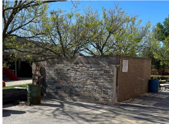
Mock Retaining Wall
