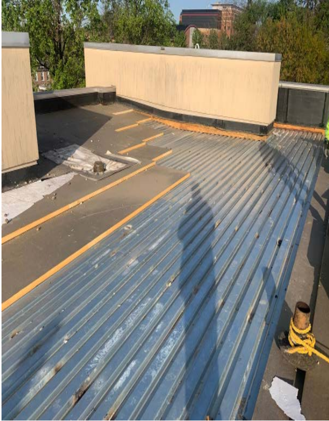
New roof board and insulation
