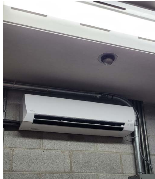
MAY 9 TH – FIRST NEW UNITS INSTALLED
