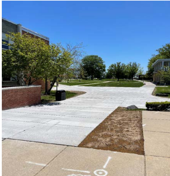
Concrete ramp at the Quad
