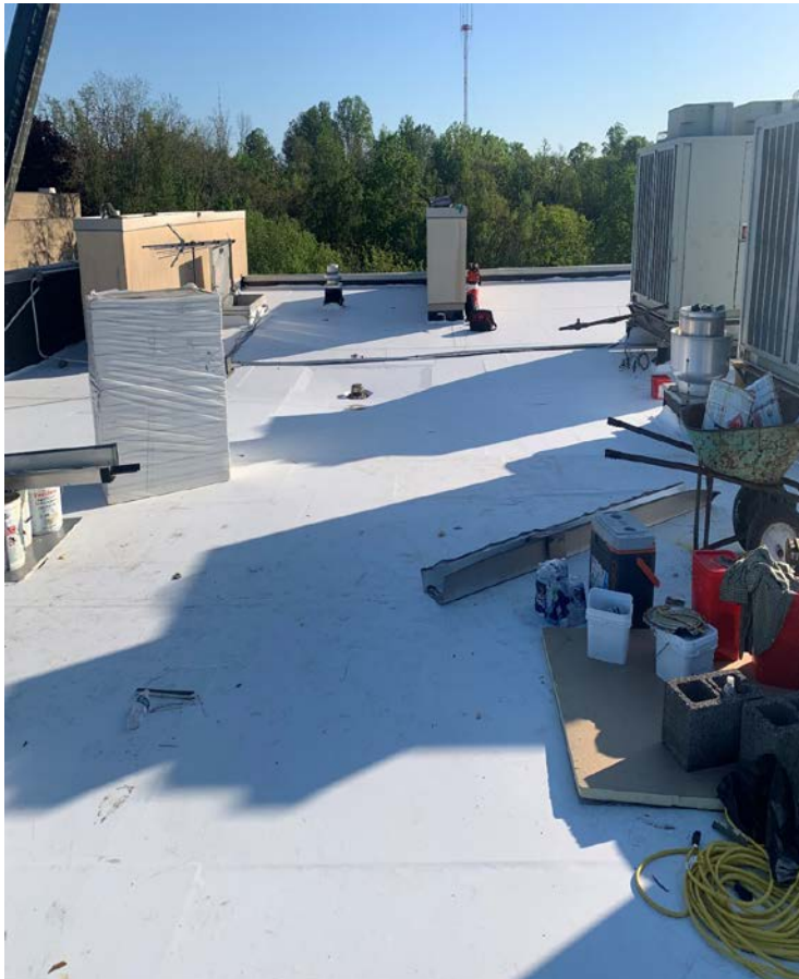
New energy efficient roof – TPO
